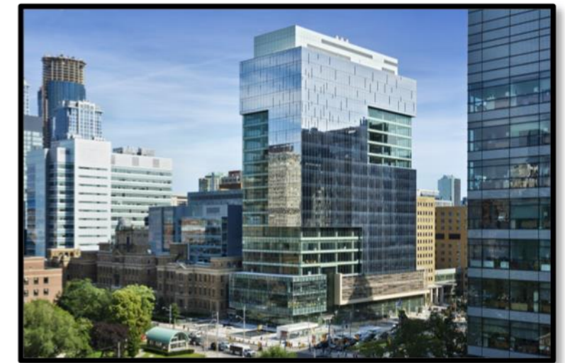
MaRS West Tower 661 University Avenue
